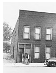
PROPERTIES DEMOLISHED FOR RYAN EXPY.
