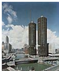
MARINA CITY TOWERS, 1965
