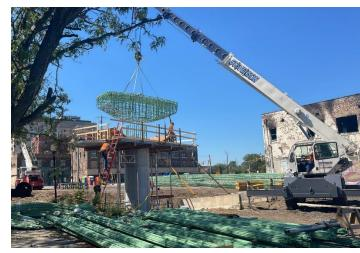
North Segment Activities: Substructure work for elevated structures including installation of bents, caissons, piers, and foundations
