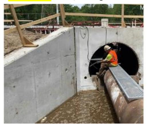
Installing final detail at Weiland Ditch culvert - wildlife shelf
