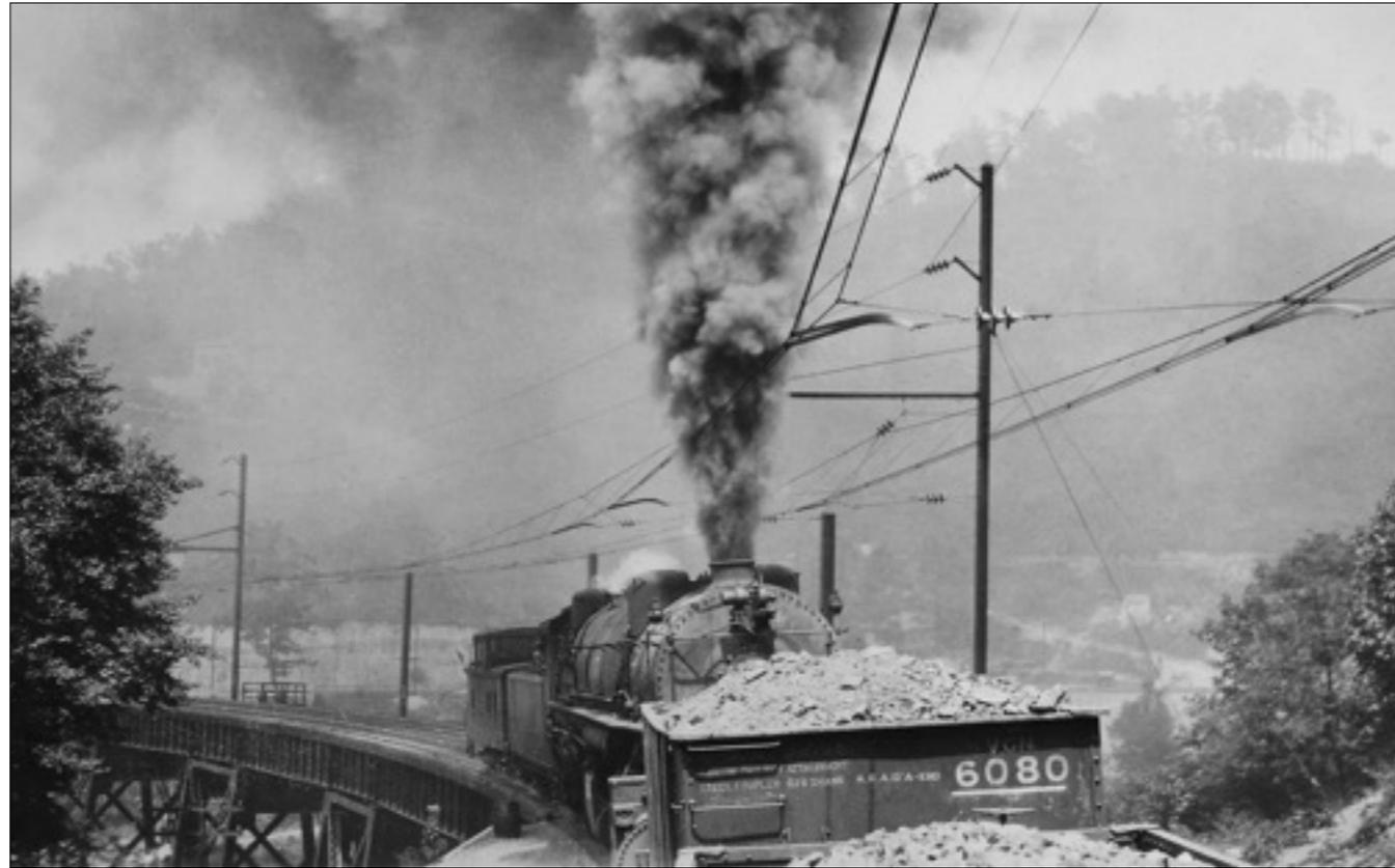
Eidenbenz also traveled extensively in the U.S., photographing trains wherever he went. That include a trip to southern West Virginia, where he rode atop a loaded coal car on the Virginian Railway. The Virginian electrified its crossing of the Alleghenies in the late 1920s—the wires are up in this image, but not yet turned on. Pushing Fred’s train is one of the railway’s massive 2-10-10-2 articulated steam locomotives.
